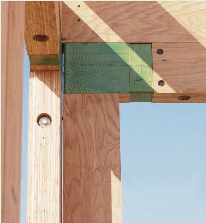
Photos above & lower left & lower right : KEYLAM® Earthquake-Resistant Portal Frame in construction
